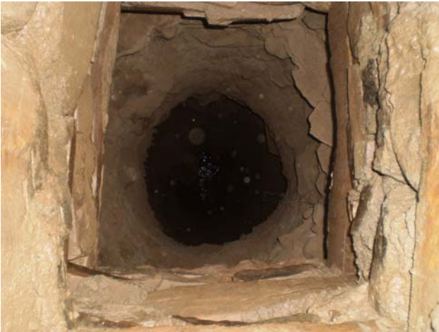
Inside of the shaft
