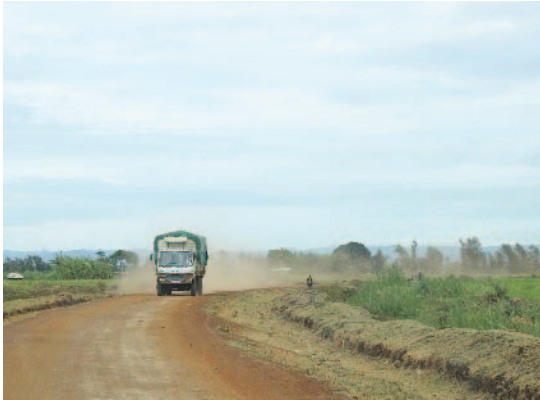
Photo19 Unsurfaced road in the scheme. Many transporting track vehicles use the road. But heavy rain makes tracks sink into the mud easily.
