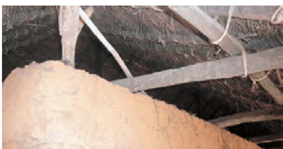
Photograph 3-1-30: Trunks used for poles and beams of buildings
