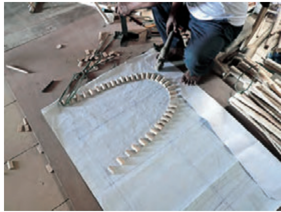
Photograph 3-2-9 Formwork production process
