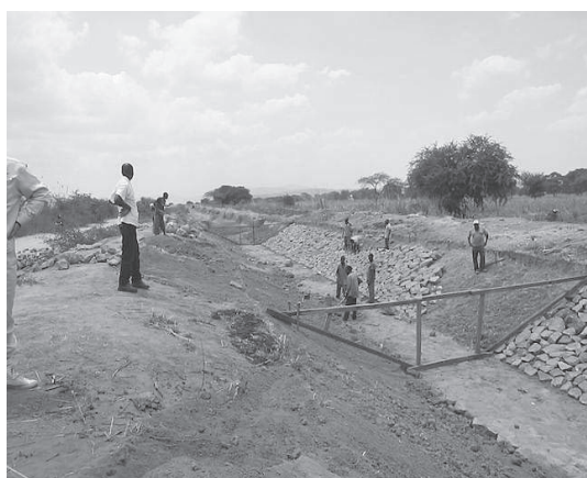
Photo II.1.18 lining work on a canal built from reserve
