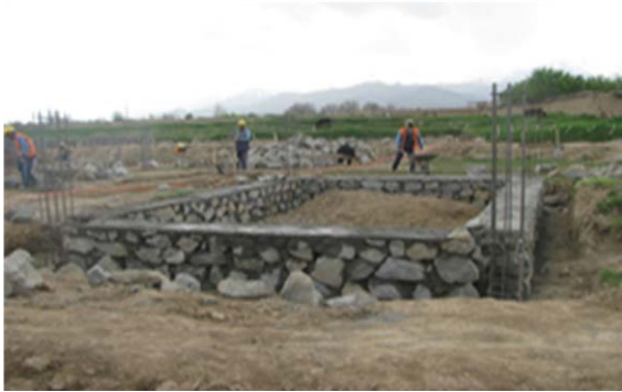
Stone masonry work of buildings foundation
