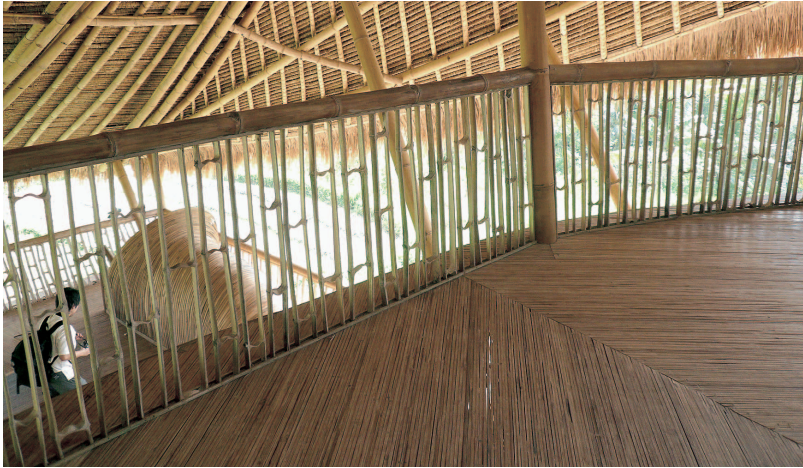
Photograph 3-2-11 Railing of Green School in Bali. Such a design as this that utilizes the cross section (torn vertically) brings out the feature of curved bamboo.
